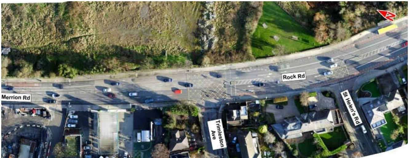
Image 5.18: R118 Rock Road / Trimleston Avenue Junction
