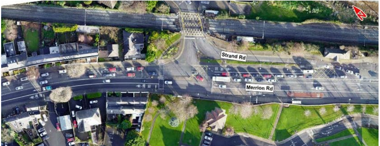
Image 5.21: R118 Merrion Road / R131 Strand Road Junction
