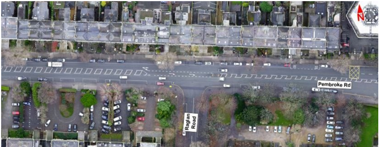
Image 5.38: R816 Pembroke Road / Raglan Road Junction
