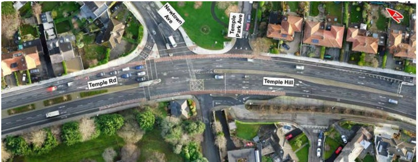
Image 5.3: R113 Temple Hill / Temple Road / Newtown Avenue Junction
