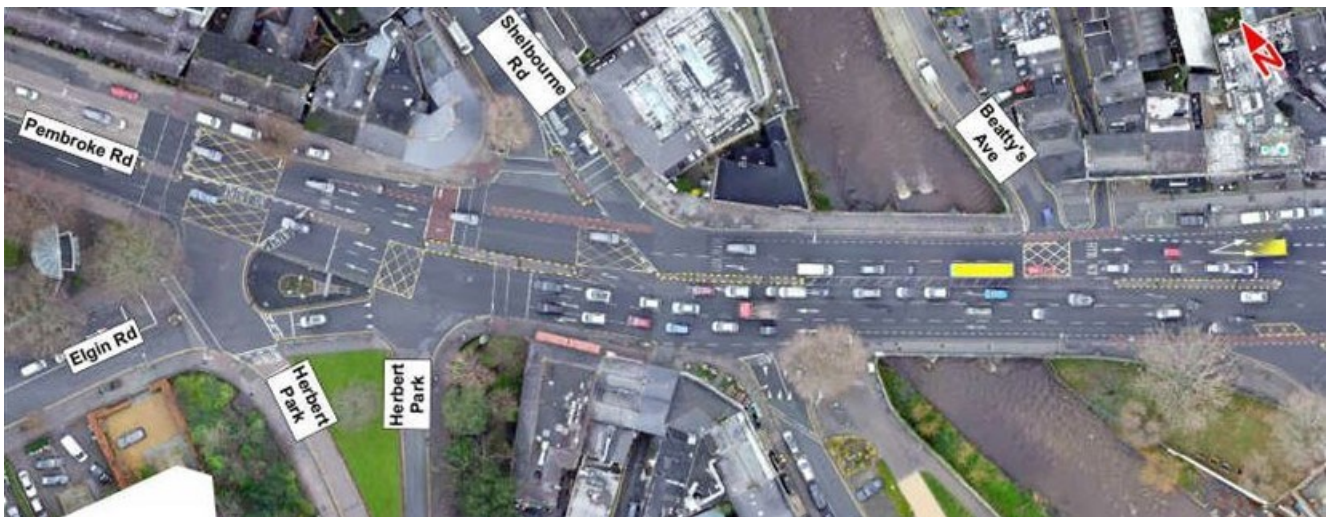
Image 5.35: R118 Pembroke Road / R815 Shelbourne Road / Herbert Park Junction
